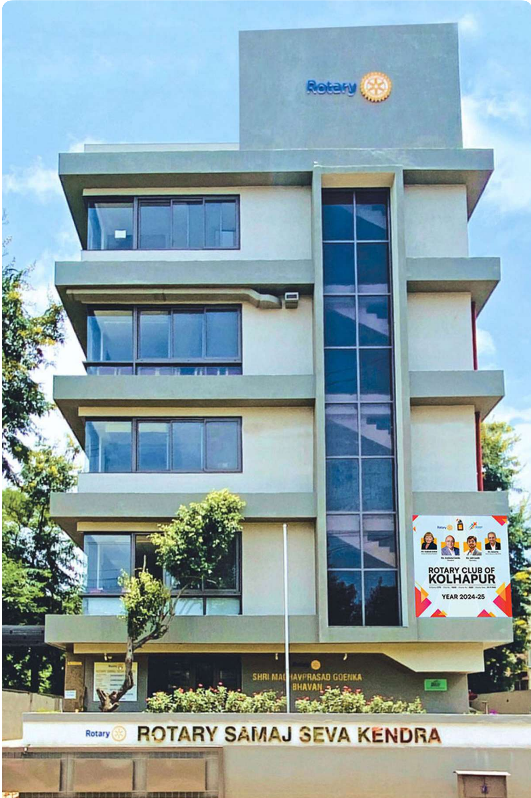
ROTARY CLUB OF KOLHAPUR'S ROTARY SAMAJ SEVA KENDRA BUILDING
